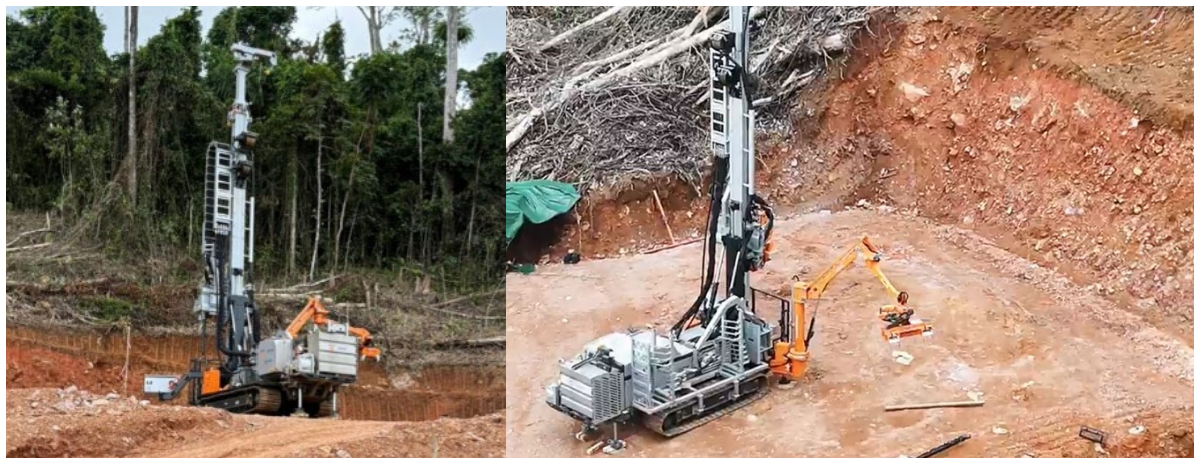
Photos: Newly arrived Rig 2 set up on the Kasie Ridge target.
