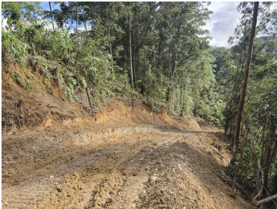
Figure 8: Newly cleared access track advancing south into the South Zone, opening the southern section of the corridor to systematic exploration.
